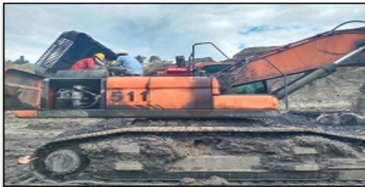
Figure 4.1 Doosan 500 LCV Excavator Repair Process
