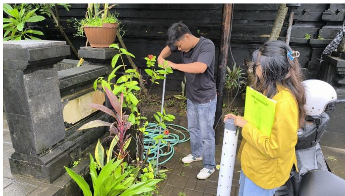
Figure 4. Biopore Installation Process
